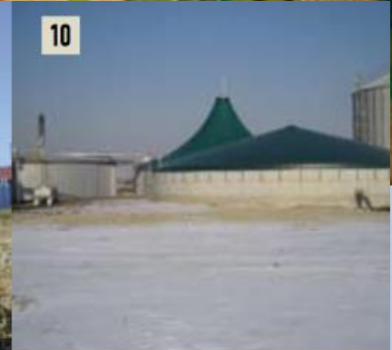
Photo 9: General view of a 2-step energy crop digestion plant with digester 1 (right) and combined gas collector and digester 2 (left)
