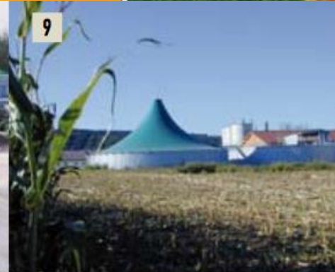
Photo 9: General view of a 2-step energy crop digestion plant with digester 1 (right) and combined gas collector and digester 2 (left)
